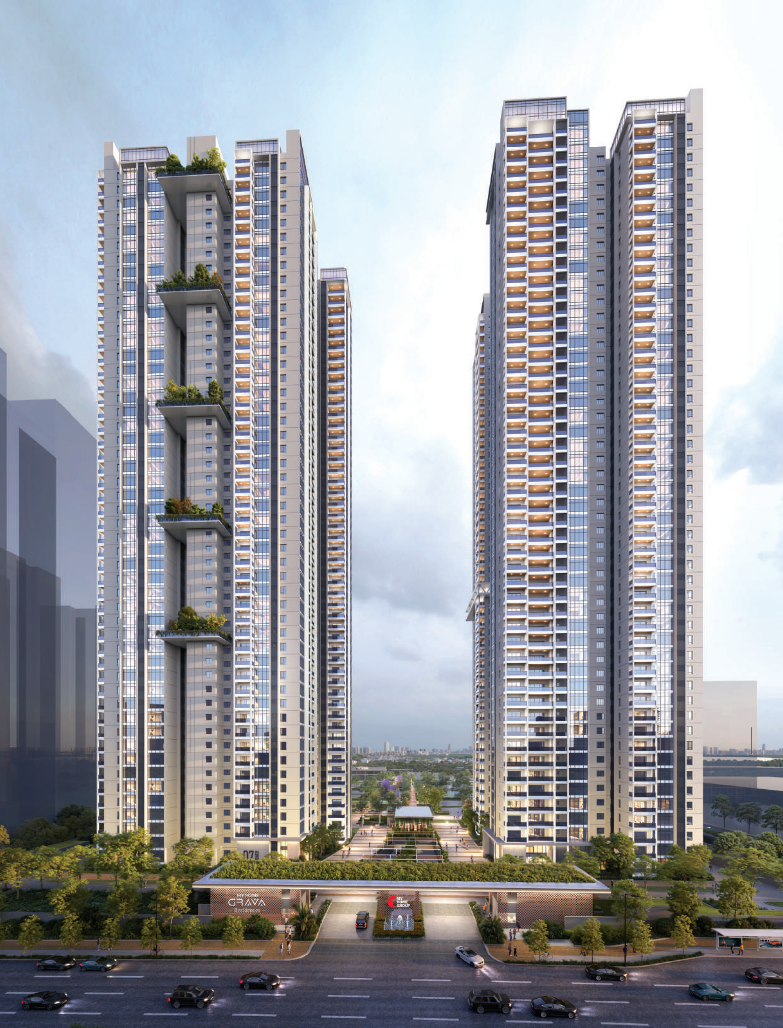
Towers, North View
