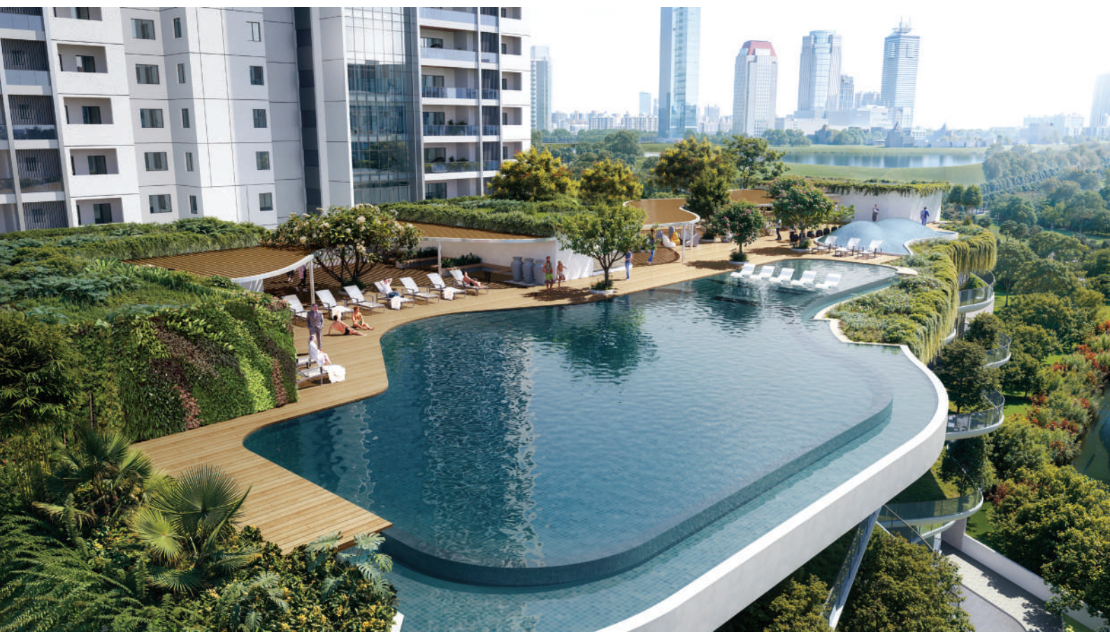
Temperature Control Swimming pool on Clubhouse Terrace
