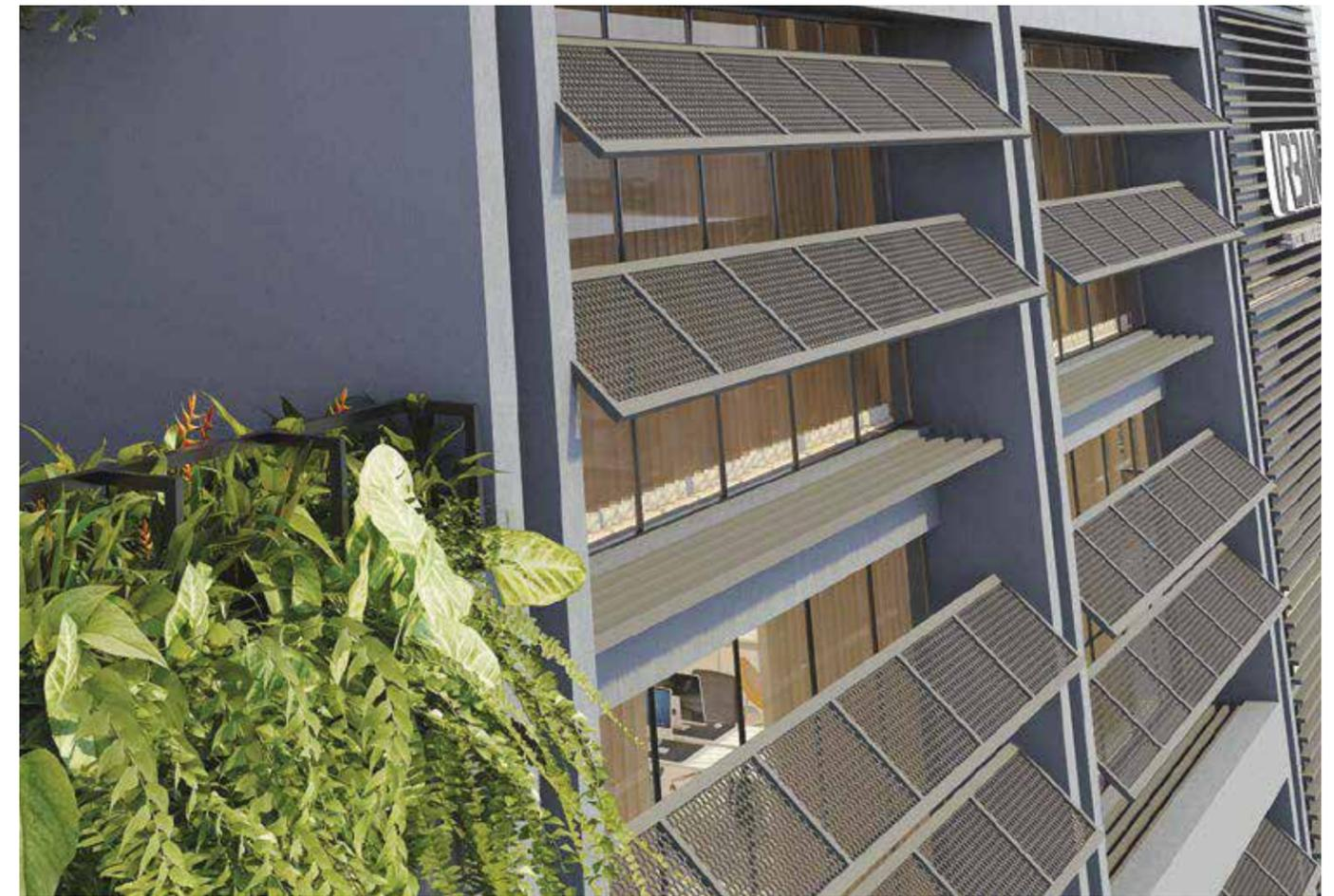
The double skin facade and substantial presence of vegetation further reduces heat loads.
